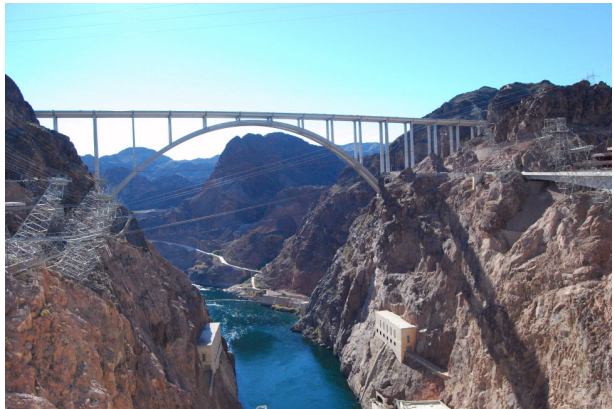
Hoover Dam Bypass Bridge, officially the Mike O'Callaghan-Pat Tillman Memorial Bridge
